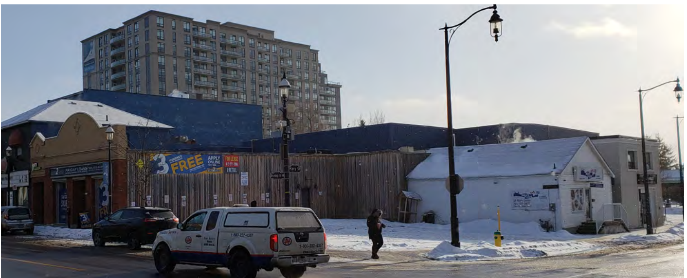
Figure 23: View of site from the north, corner of Dunlop Street West and Mary Street
