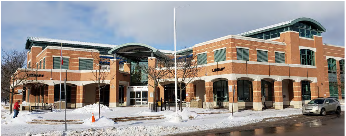
Figure 20: Barrie Public Library from Worsley Street
