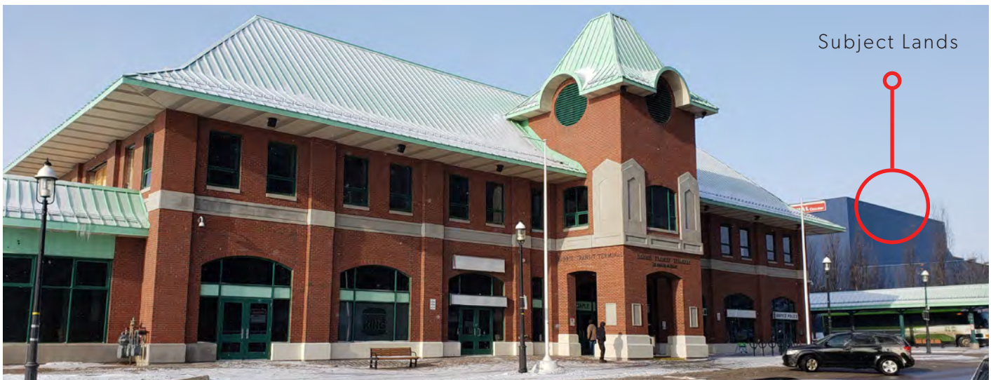
Figure 18: Photograph of existing Barrie GO Transit Terminal with subject lands visible
