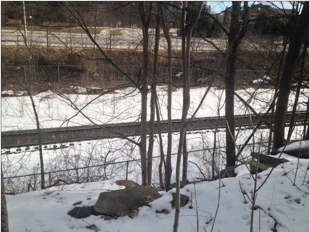
Photograph 5. View of rail corridor and Hurst Drive (Northeast) (January 2018).
