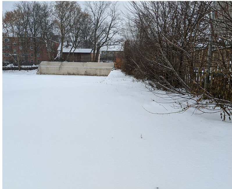
Photo 2: Facing south, remnant of southern and western building wall at 45 Penetang Street
