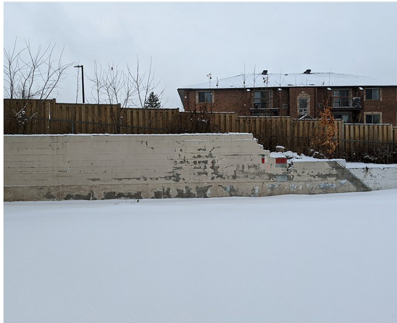
Photo 8: Facing west, remnant of western building wall at 45 Penetang Street
