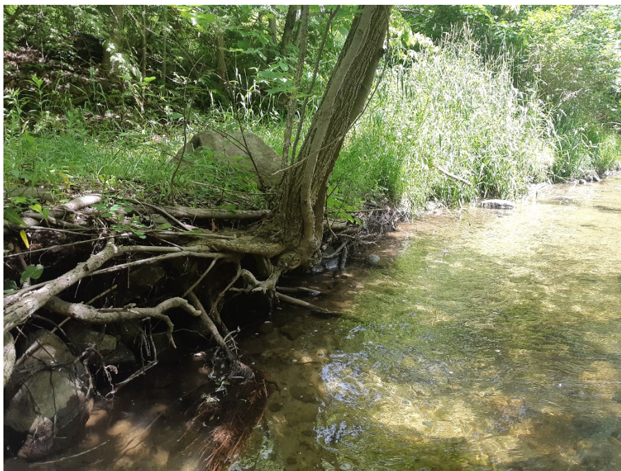
Photo 4 Undercut banks, June 2021.
