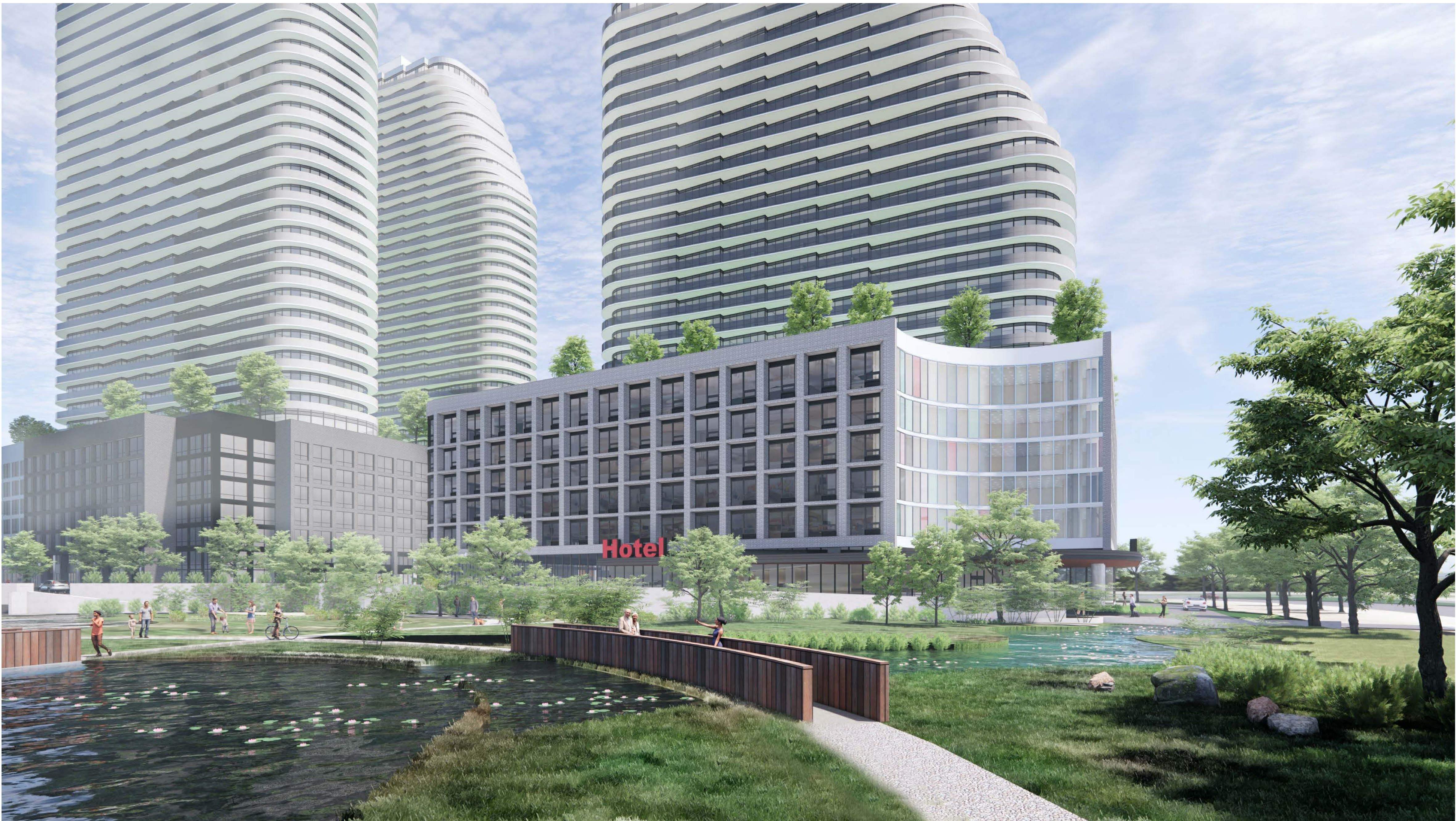
VIEW FROM OPEN SPACE LOOKING NORTH
