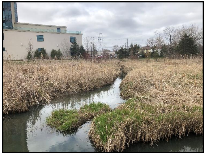
Photograph 4. (Photo Location 3) Upstream view of stormwater outlet channel (south side of creek).
