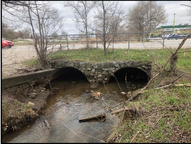
Photograph 9. (Photo Location 8) Upstream view of Bradford Street crossing.
