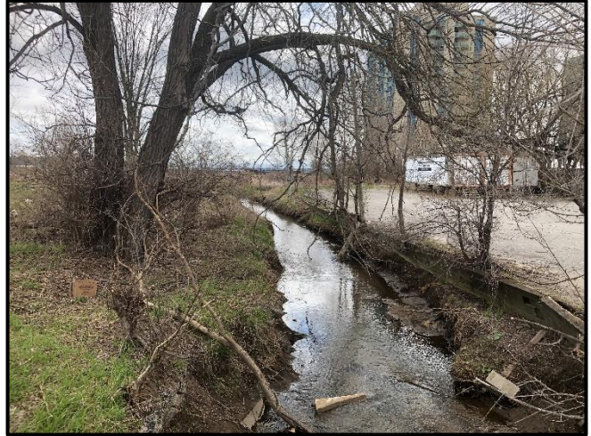
Photograph 10. (Photo Location 8) Downstream view of general conditions from Bradford Street Crossing.
