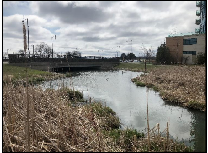
Photograph 2. (Photo Location 2) Downstream view towards Lakeshore Drive crossing.
