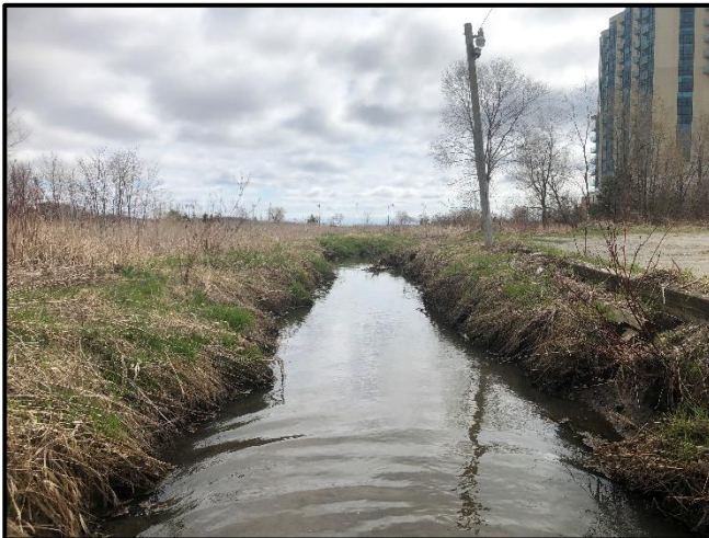
Photograph 7. (Photo Location 6) Downstream view of general conditions within corridor and evidence of active bank erosion (photo right).
