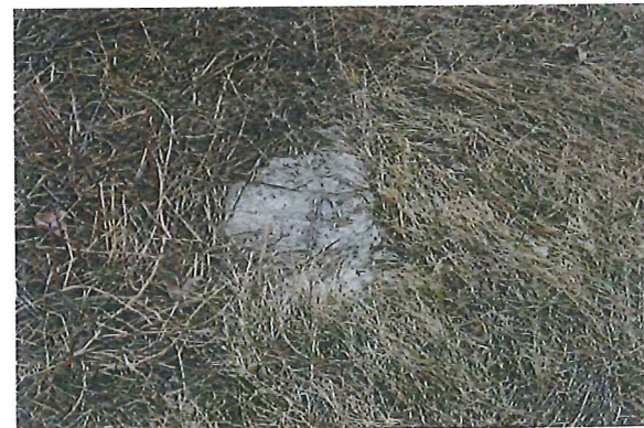
Plate 16 In-Ground Cement Fragment South of Condominium facing North
