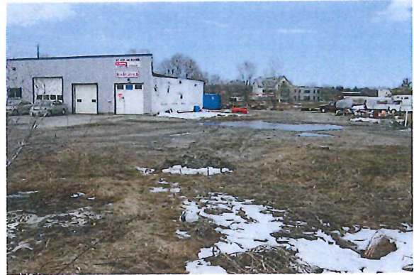
Plate 12 South and East Façade of Carsmart (75 Bradford Street) and Ground Conditions facing North
