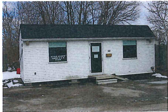
Plate 8 North and West Façade of 55 Bradford Street facing Southeast
