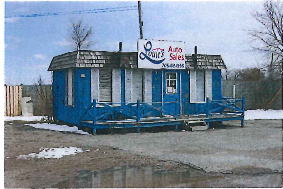
Plate 6 North and West Façade of Louie's Auto Sales (51 Bradford Street) facing Southeast
