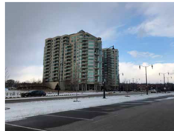
Figure 37. Existing Grand Harbour Condos to the north
