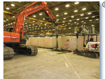
④ Deep soil mix columns (shown) and mass soil mix cap constructed for settlement control of new tanks in Louisiana.
