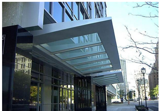
Figure 3.9 Examples of wind mitigation measures
