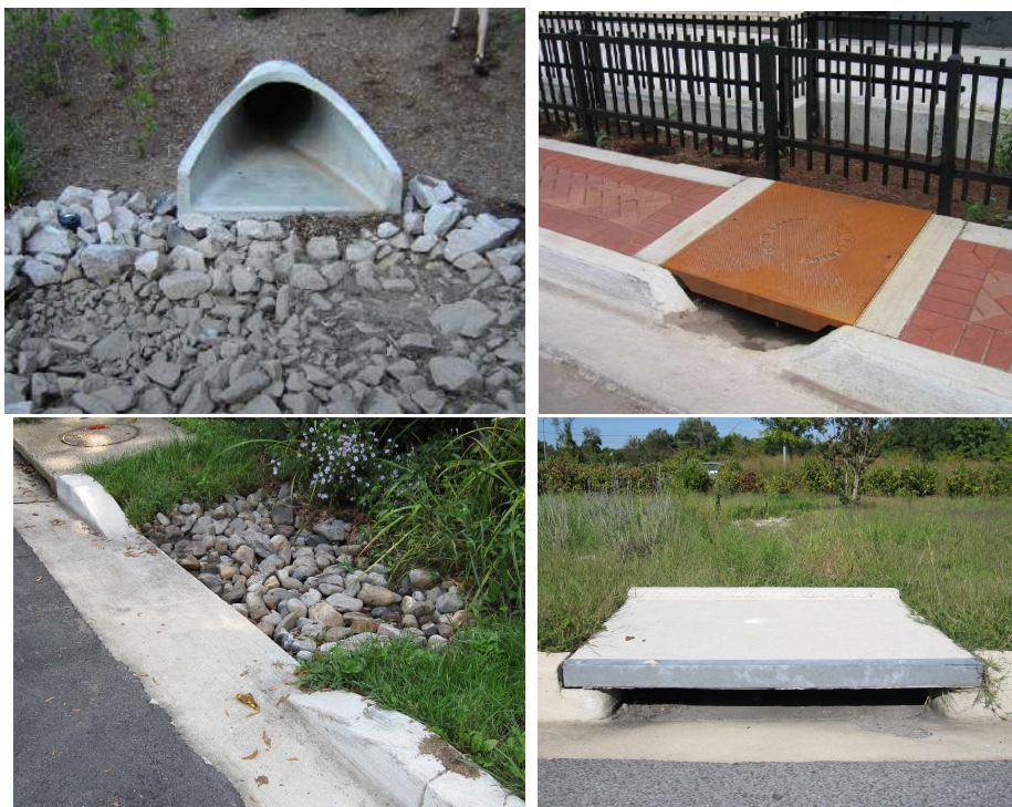
Figure 4.5.10 Examples of inlets to bioretention practices
