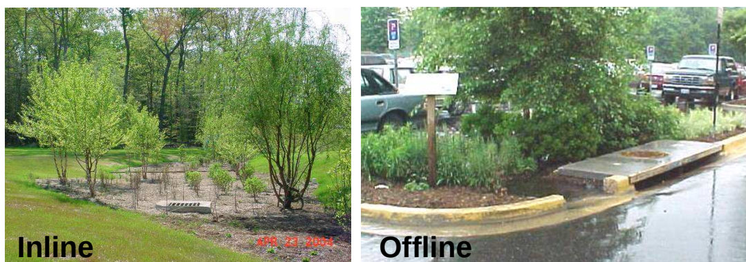
Figure 4.5.9 Examples of inline and offline bioretention
