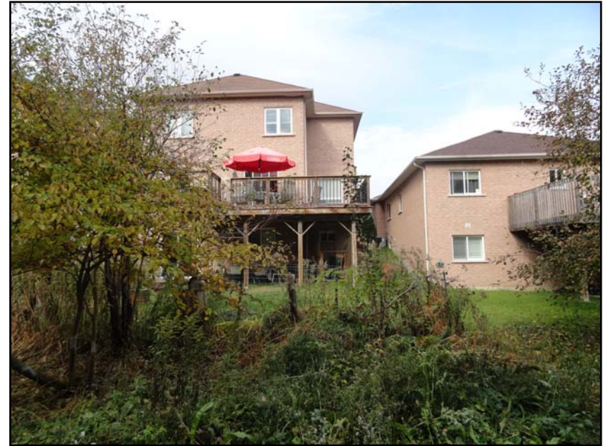
Photograph 6. View of as-built residential lots (2 storey brick dwellings), part of south side of Loon Avenue subdivision, that abuts the property to the north
