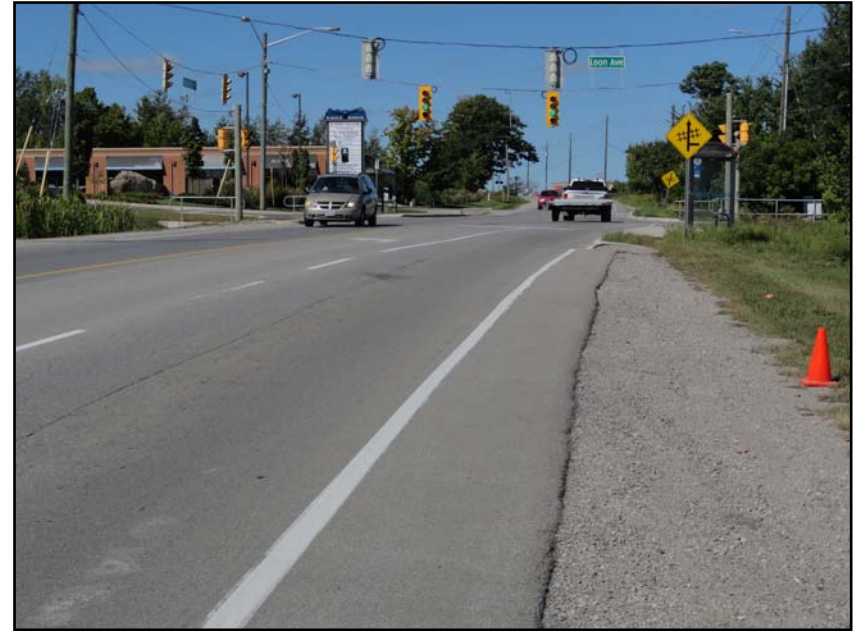
Photograph 2. Northward view of Huronia Road and signalized intersection with Loon Avenue
