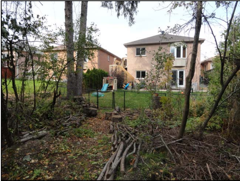
Photograph 5. View of as-built residential lots (2 storey brick dwellings), part of south side of Loon Avenue subdivision, that abuts the property to the north
