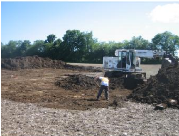
Plate 3. Stage 4 Topsoil Stripping of the Wice Site (BcGv-37) (view northeast)
