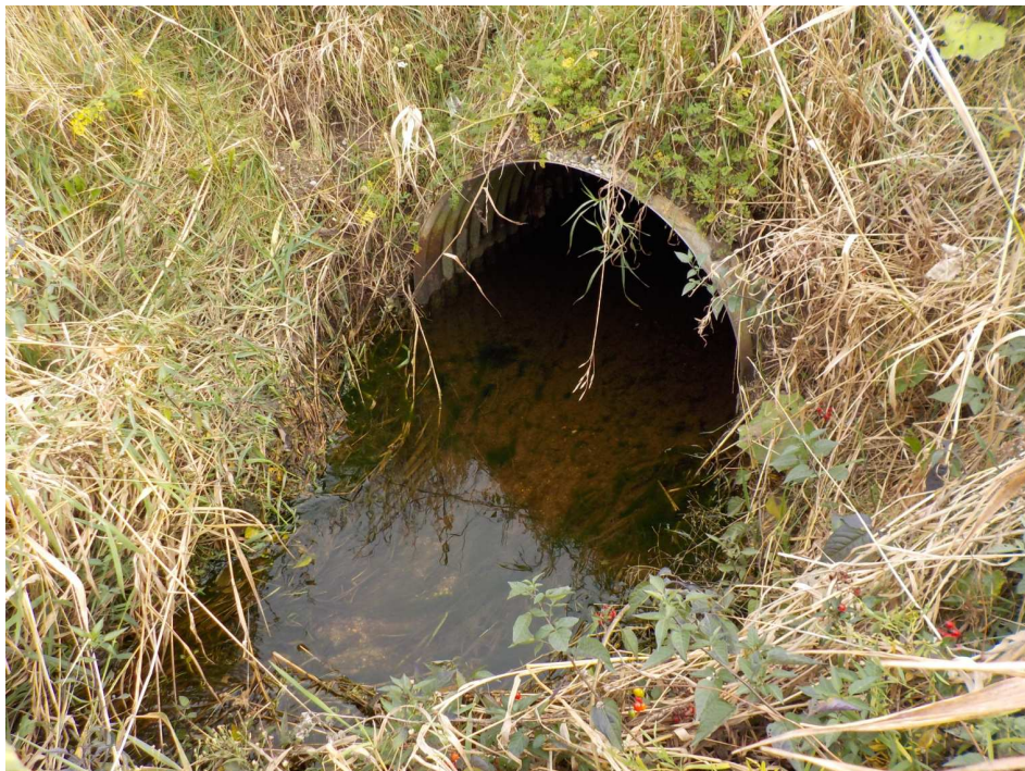
Photograph 14: Tributary of Lovers Creek at Lockhart Road CSP culvert outlet (facing south; October 25, 2017).
