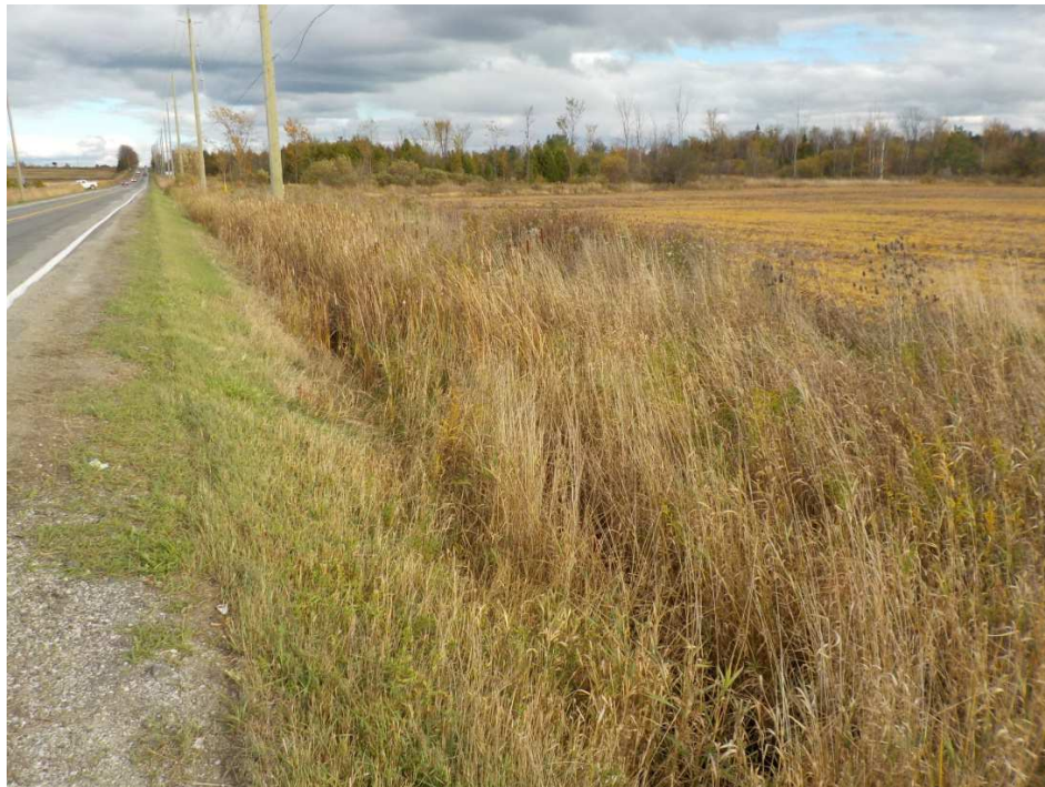
Photograph 16: Drainage Ditch C on south side of Lockhart Road (facing east from CSP culvert inlet); October 25, 2017).
