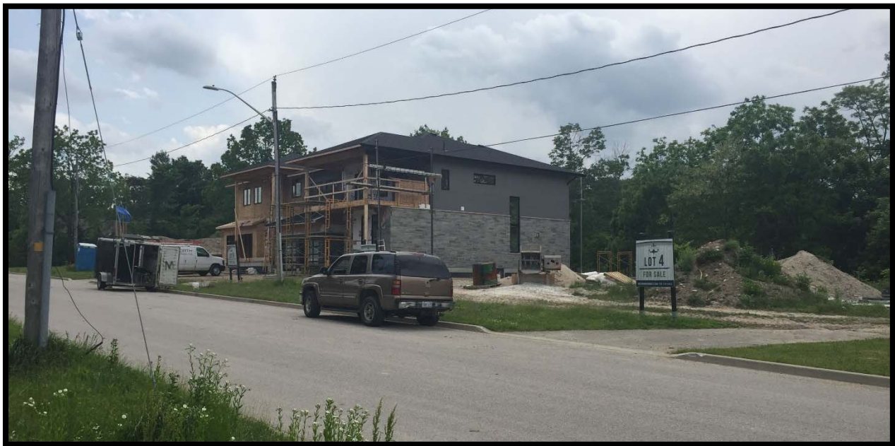
Figure 7: Adjacent Properties Under Construction & Lots for Sale
