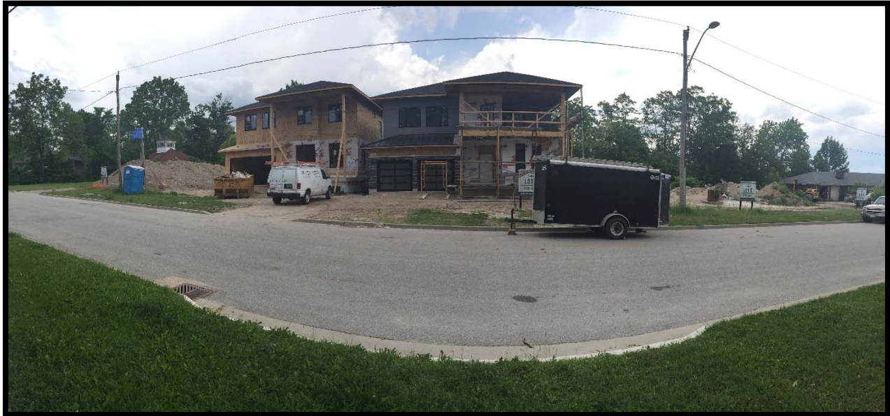
Figure 6: Adjacent Properties Under Construction – 400 to 408 Cox Mill Road
