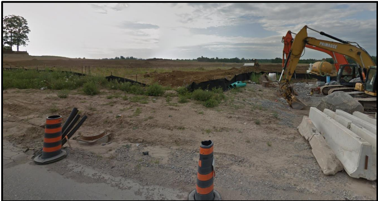
Figure 3. Site Alteration undertaken on Lands owned by GG(9 Mile)
