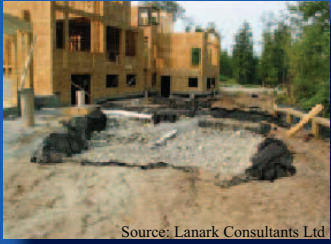
Source: Lanark Consultants Ltd.
