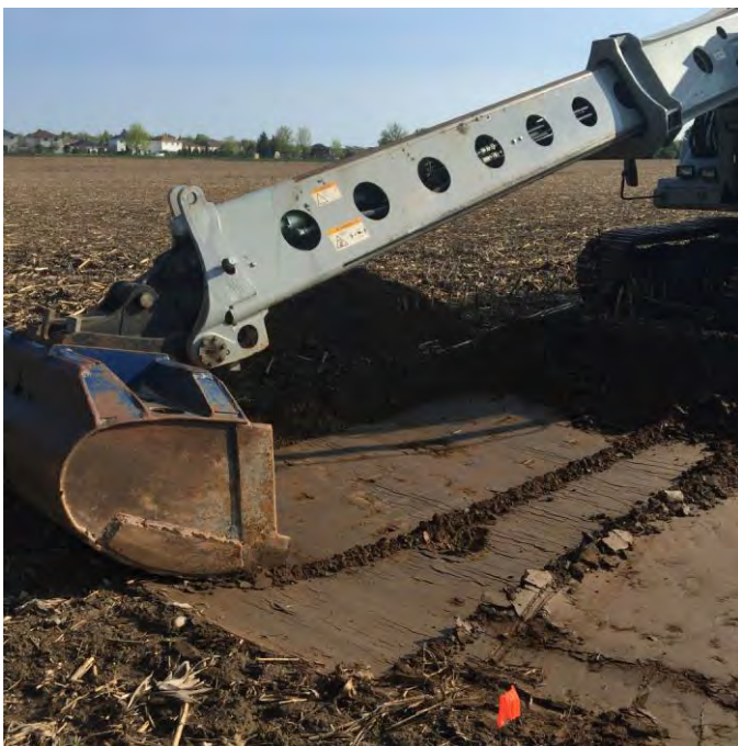
Plate 3: Initial Gradall excavation.
