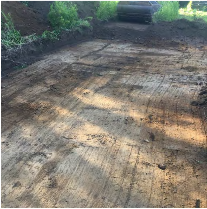
Plate 1: Mechanical topsoil removal.
