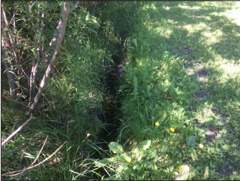
Photograph 17. Upgradient view of man-made drainage swale, along south edge of existing as-built lot that fronts onto Highway 27, and which conveys surface runoff from the highway, eventually draining into the Bear Creek tributary
