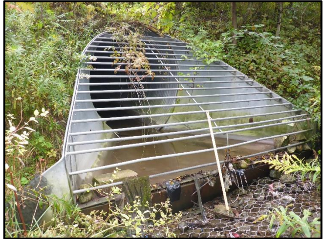
Photo 18 (Photo Location 21) Reach BEA2-7 Upstream view of Loughheed Road culvert and gabion drop structure.
