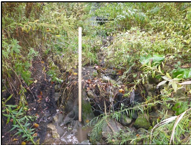
Photo 19 (Photo Location 22) Reach BEA2-7 Upstream view at downstream transition of gabion gabion drop structure.
