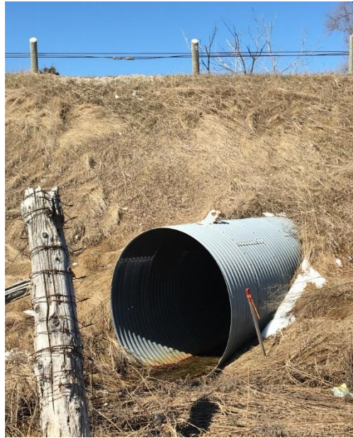
Photo 11. View of the culvert located in the northwest side of the Phase One Property.
