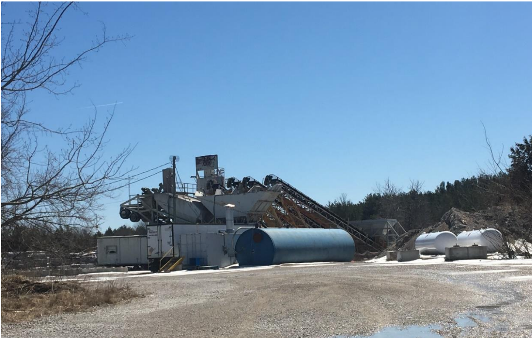
Photo 20. View of concrete plant located in the southeast portion of the Phase One Study Area at 4165 Salem Road (looking southeast).
