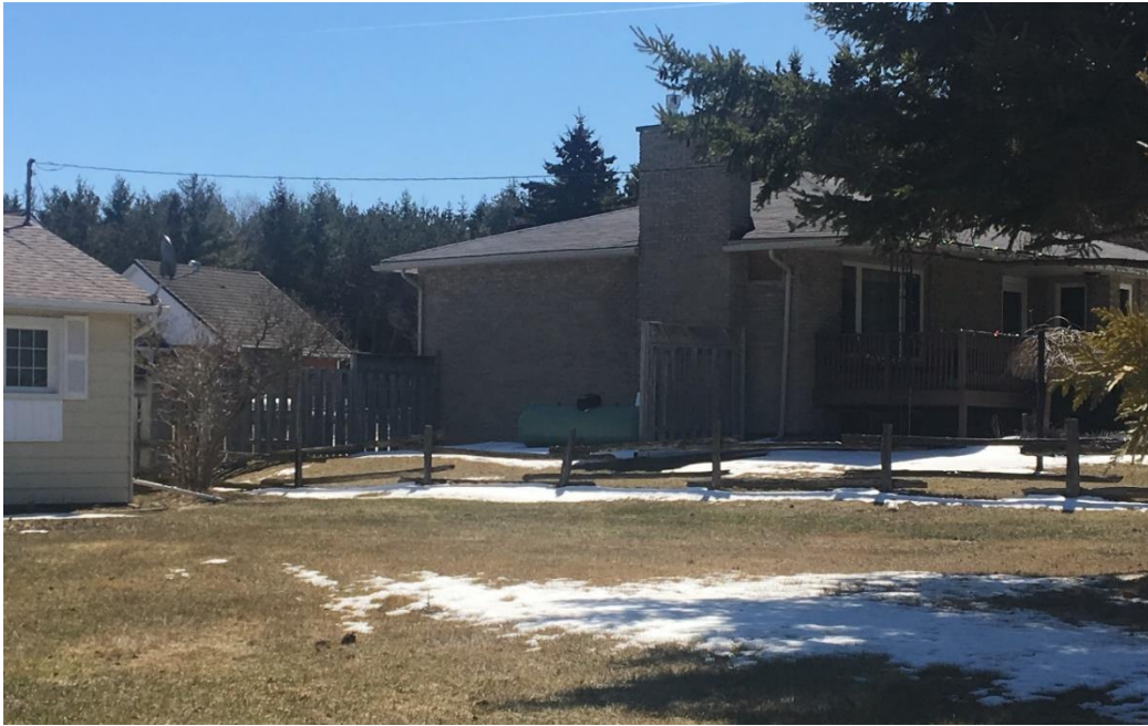
Photo 23. View of the oil storage tank located in the southwest portion of the Phase One Study Area at 7975 County Road 27 (looking southeast).
