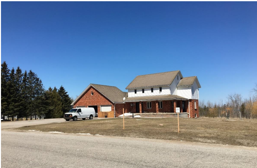
Photo 16. View of the south adjacent property to the Phase One Property. Residential house at 500 Salem Road (looking northwest).
