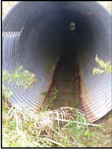
Photo 9 (Photo Location 14) Reach BEA1-4 Downstream view of CSP (1250 mm) under County Road 27.
