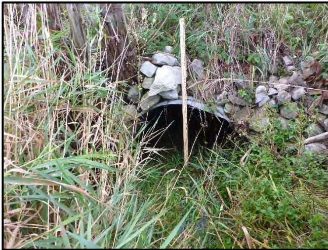
Photo 11 (Photo Location 10) Reach BEA1-4 CSP (750 mm) under informal crossing.
