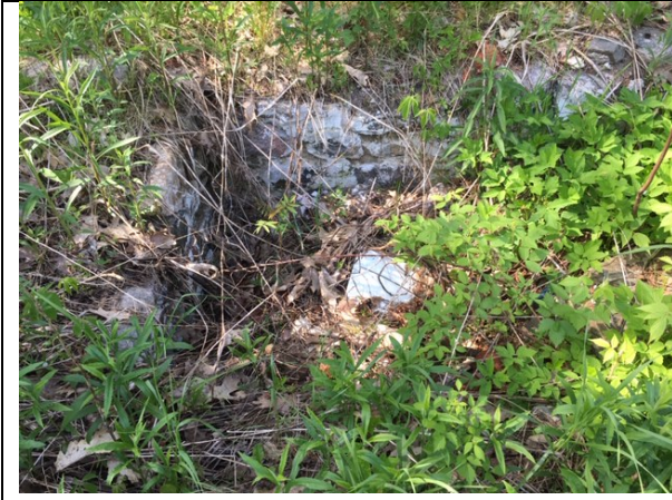
IMAGE 1 MODERN FOUNDATION RUINS
