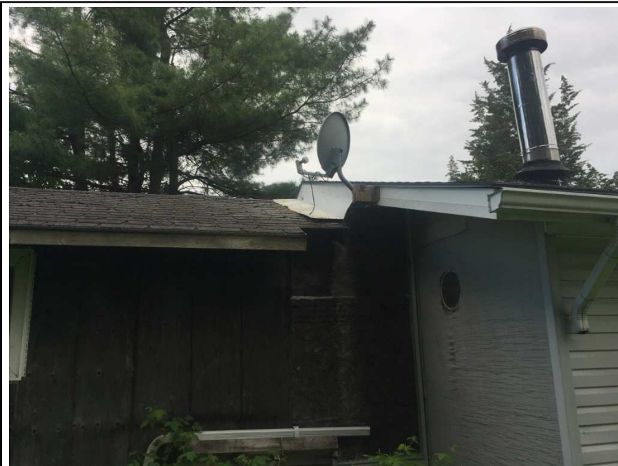
Photograph 4. No holes or spaces which bats may utilize to access the interior of the garage were noted. The chimney on the garage is capped and thus does not provide habitat for Chimney Swift (May 31, 2017).
