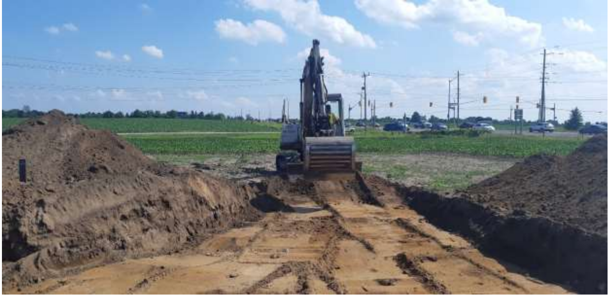
Image 5: Mechanical Excavation in Progress. Facing Southwest.
