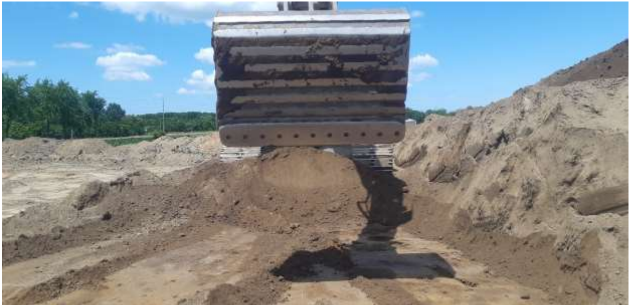
Image 6: Mechanical Excavation in Progress. Facing Northwest.
