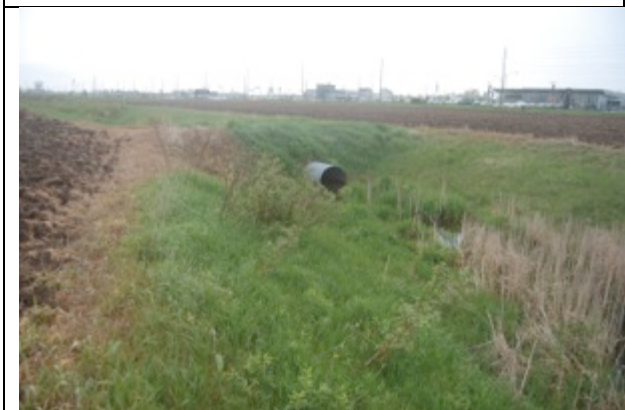
PLATE 29 STREAM CULVERT AND STEEP SLOPE EMBANKMENTS
