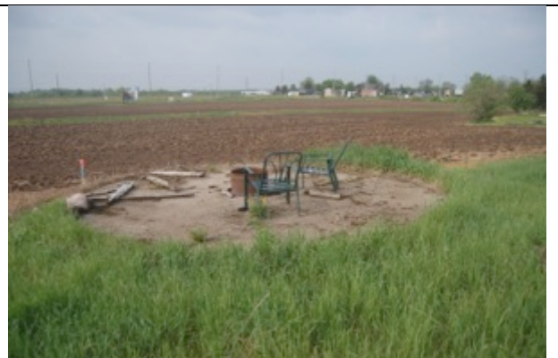
PLATE 16 CONCRETE SILO PAD
