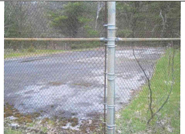
IMAGE 6 ASPHALT TENNIS COURT
