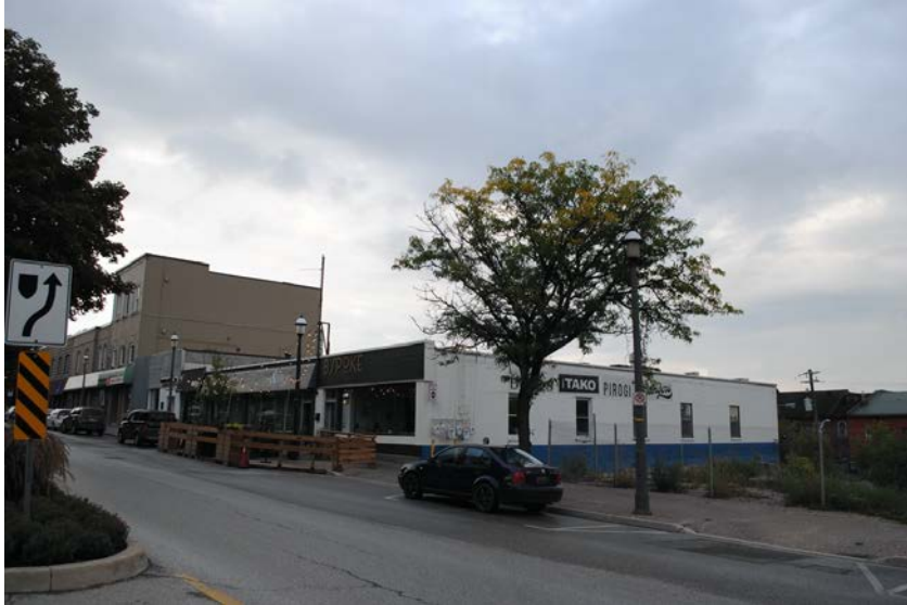
View of the northern edge of the subject site at Collier Street, looking east towards one-storey commercial structures at 55-61 Collier Street.
