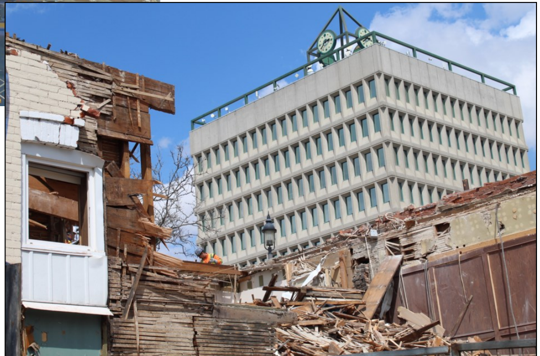
47 Collier Street during demolition in 2018. Images published in the local online news source, Barrie Today, show the building before and during demolition. It appears that the building was indeed timber with a brick facade. Source: Barrie Today.
