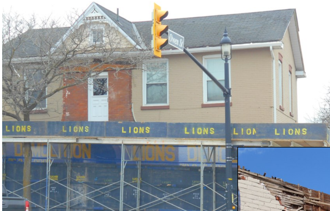
47 Collier Street during demolition in 2018. Images published in the local online news source, Barrie Today, show the building before and during demolition. It appears that the building was indeed timber with a brick facade. Source: Barrie Today.
