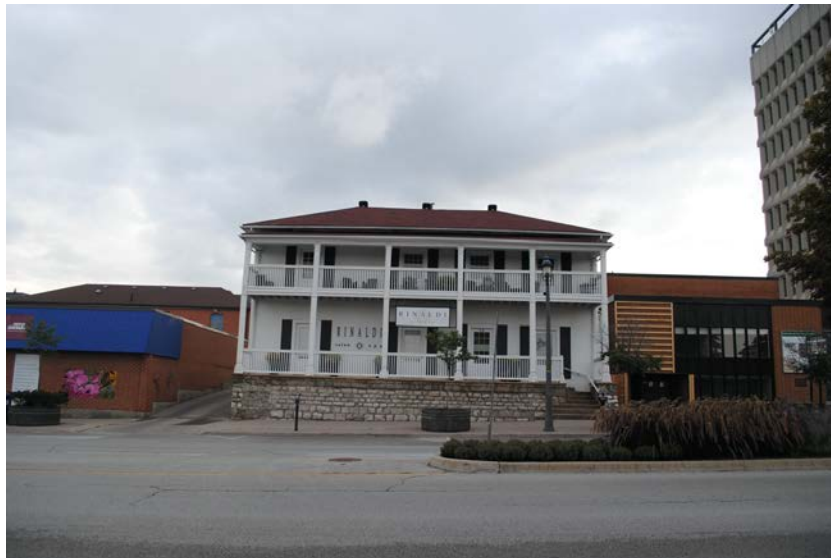
View of Collier Street, looking north from the subject site. At 58 Collier is a 2-storey hipped roof structure with balcony.
