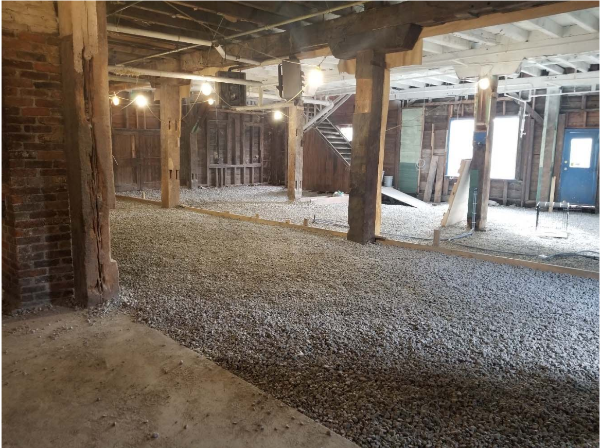
Figure 5 Looking southeast at the south side of the building, September 2022.
