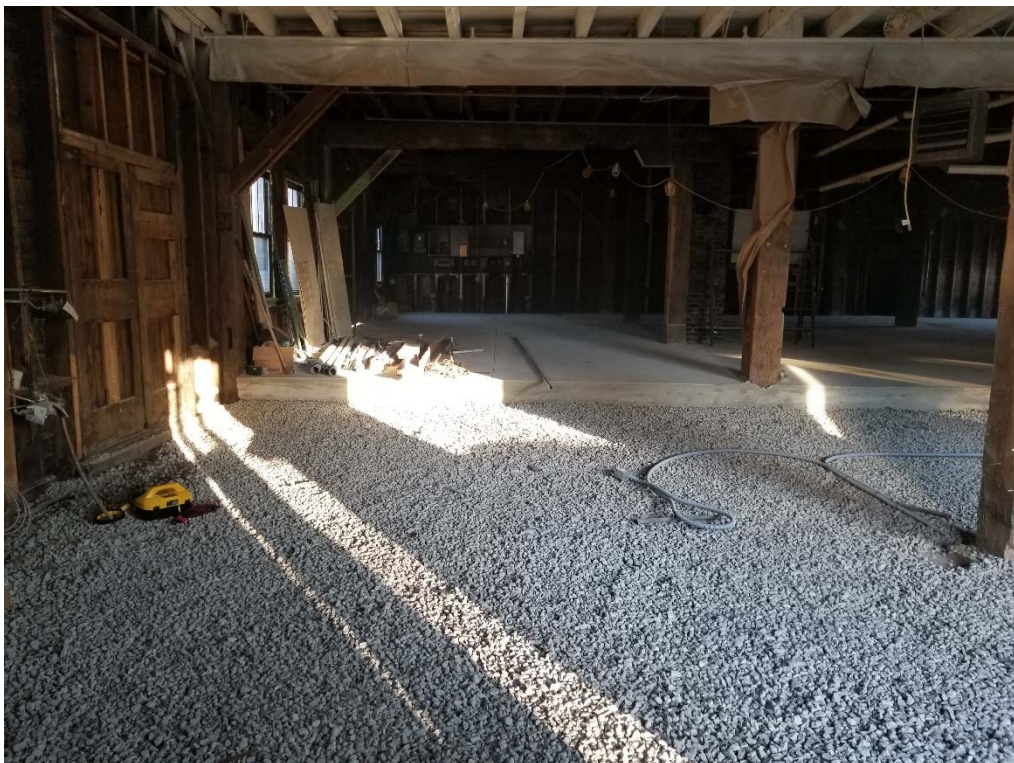
Figure 12 Looking north at the west side of the building, October 2022.
