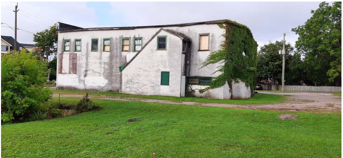
Figure 2 Looking southwest at the west side of the Site, September 2022.
