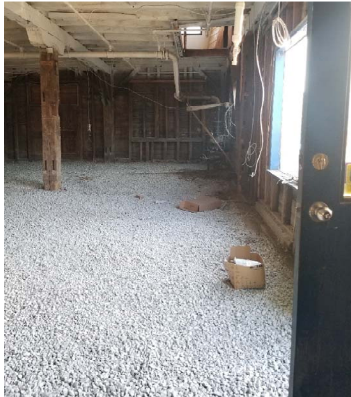
Figure 14 Looking east at the south side of the building, October 2022.
