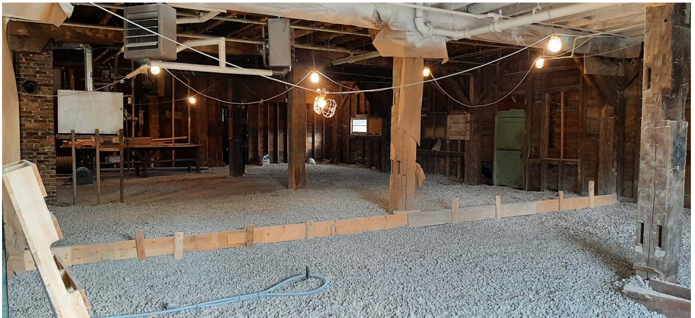
Figure 6 Looking northeast at the northeast side of the building, September 2022.
