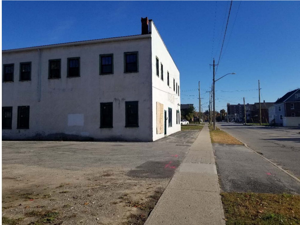
Figure 9 Looking east along the south side of the Site, October 2022.
