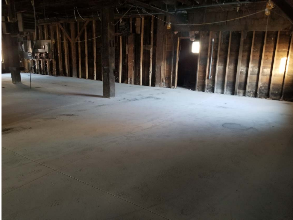
Figure 13 Looking northwest at the north side of the building, October 2022.
