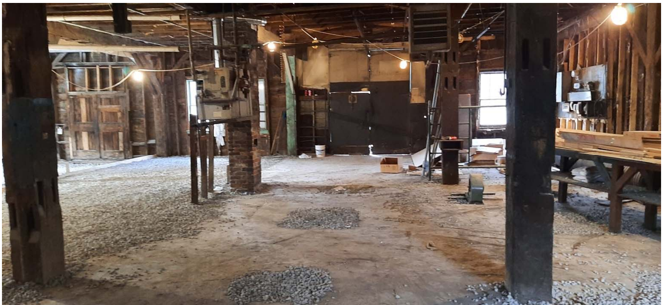
Figure 4 Looking west at the north side of the building, September 2022.
