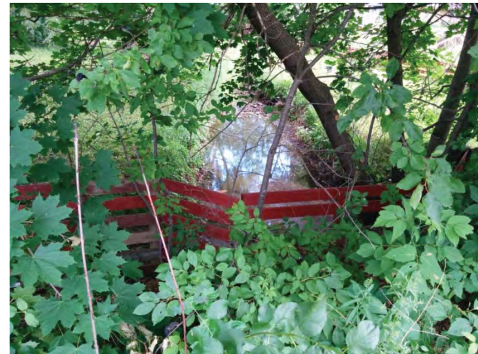
Site 7 – Sophia Creek at Davidson and Gunn (Gunn St. Culvert)
