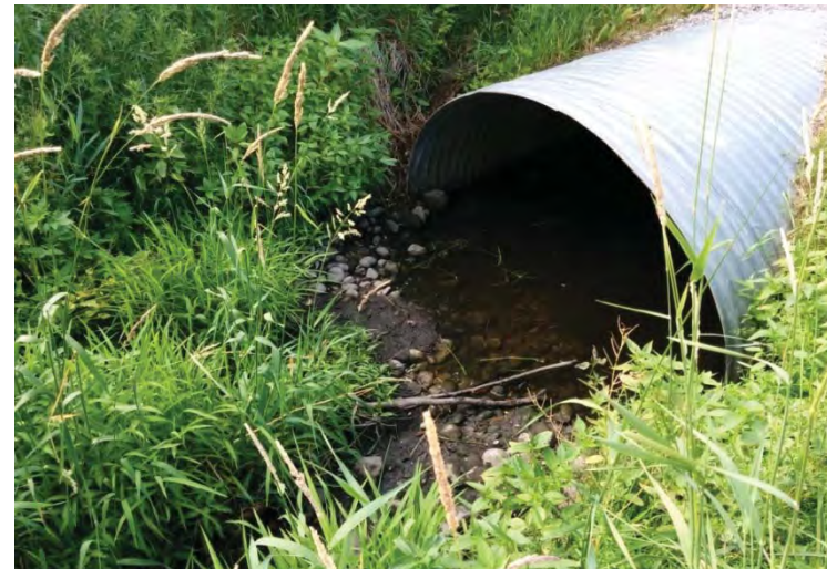
Site 4 - Sophia Creek at MacMorrison Park (Culvert)
