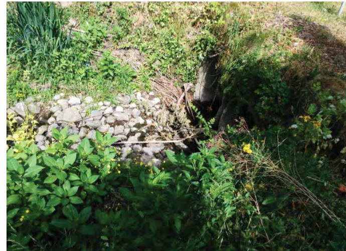
Site 5 – Sophia Creek at Davidson and Grove (Grove St. Culvert Crossing)
