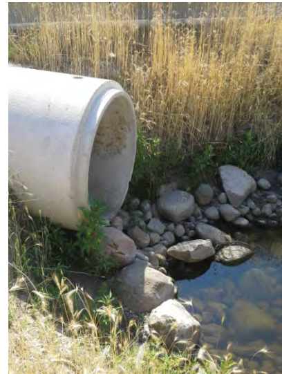
Photograph 8: Perched outlet at Bothwell Crescent crossing (Fisheries Survey Site 6).
