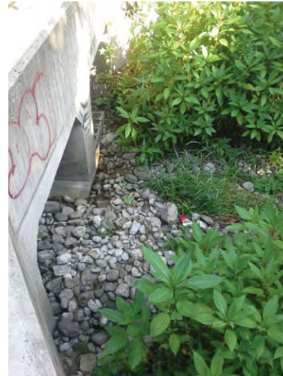
Photograph 6: Culvert inlet at St. Vincent Street (Fisheries Survey Site 5).
