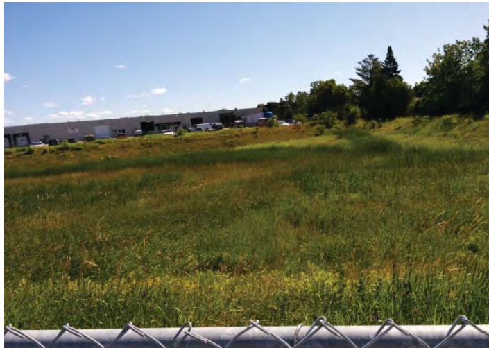
Site 10 – Ottawa Ave Stormwater Retention Pond
