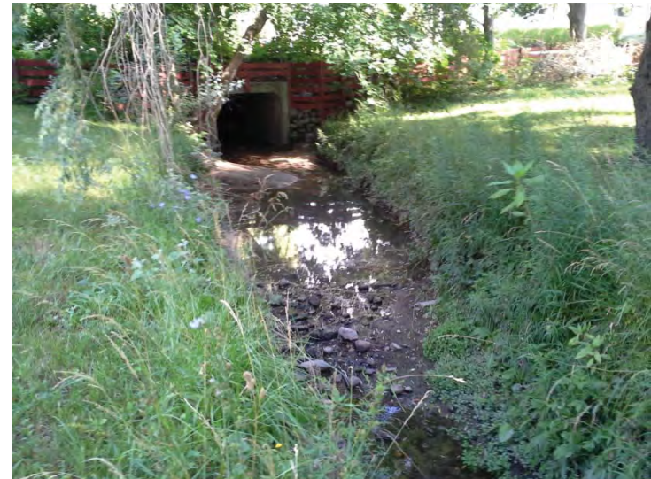
Photograph 12: Sophia Creek between Gunn Street and Berczk Street (Fisheries Survey Site 9).
