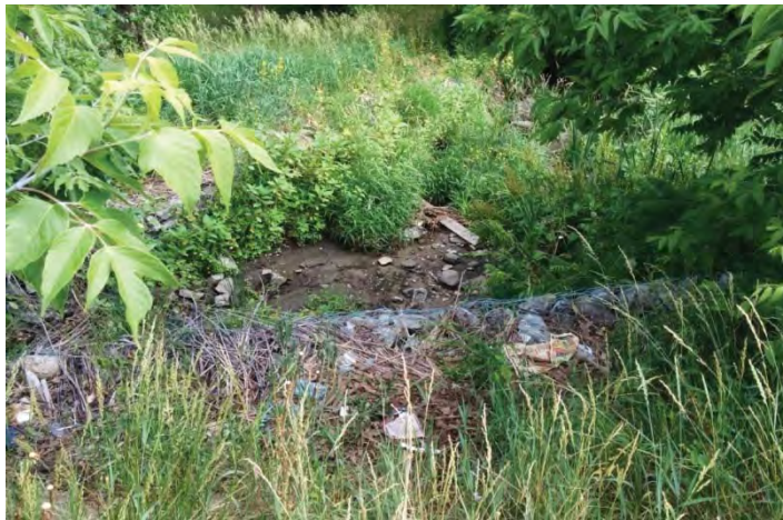
Site 6 – Sophia Creek at Parkdale and Northpark (Parkdale Culvert, Substrate/Watercourse Flow)
