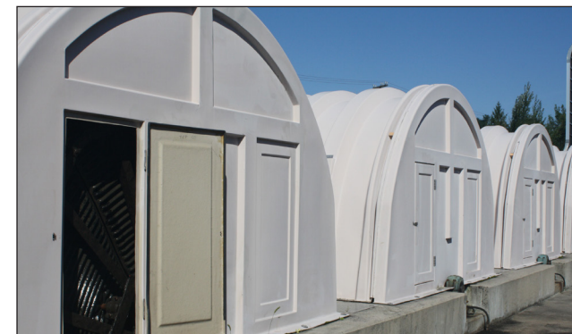
Wastewater Treatment Facility
