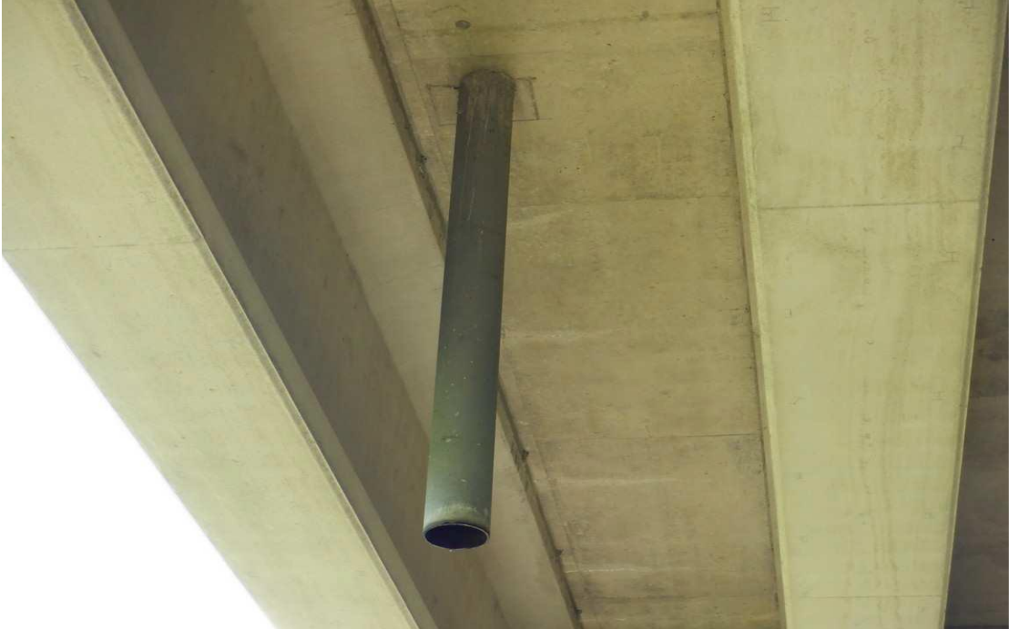
Figure 24 - Typical Bridge Condition Photo
