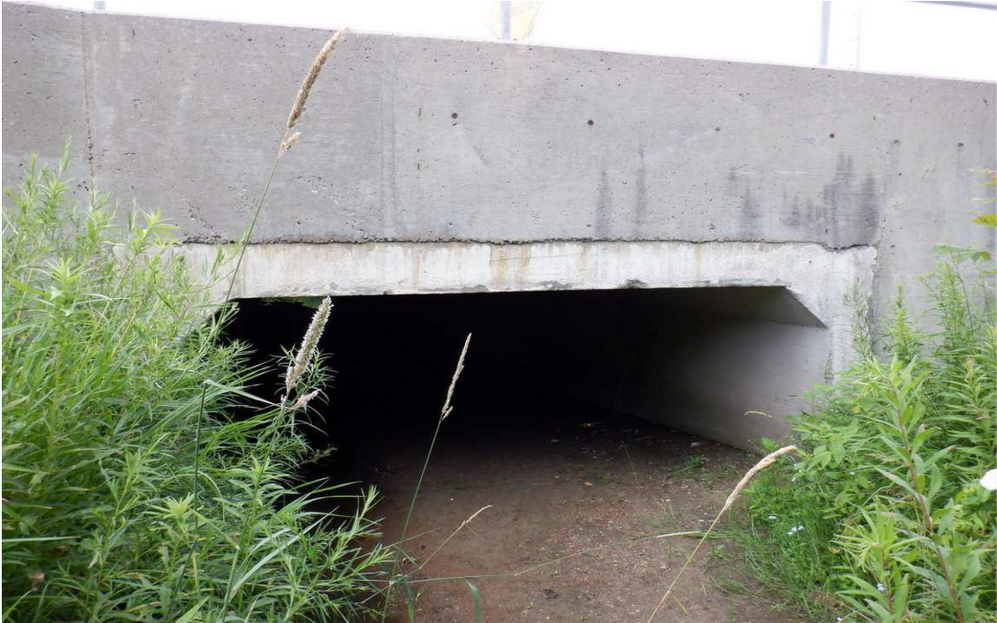
Figure 25 - Typical Bridge Condition Photo
