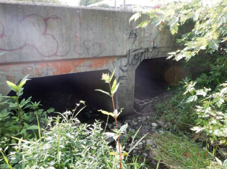
**Figure 3 – Structural Culvert in Fair Condition**
