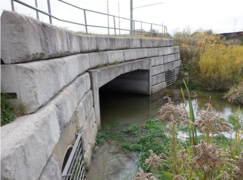
**Figure 2 – Structural Culvert in Good Condition**
