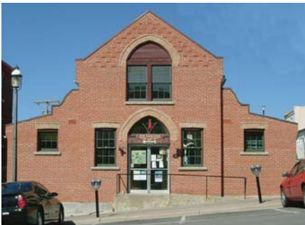
Former Armoury at 36 Mulcaster St.
