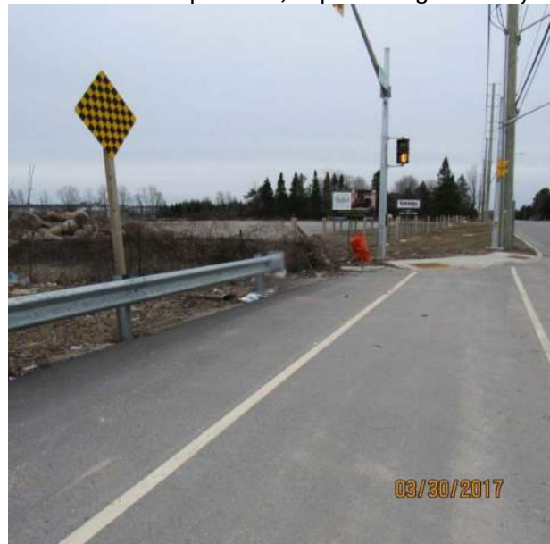
Plate 16: Southwest view on Essa Rd at Coughlin Dr.; Area is disturbed, no potential
