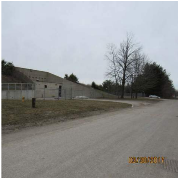
Plate 9: Northeast view of Harvie Rd; Area is disturbed, no Stage 2 required.
