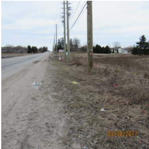
Plate 5: Northeast view on Essa Rd; Area beyond disturbed road shoulder exhibits potential, requires Stage 2 test pit survey.
