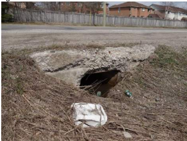
Plate 5: Concrete and corrugated steel pipe culvert.
