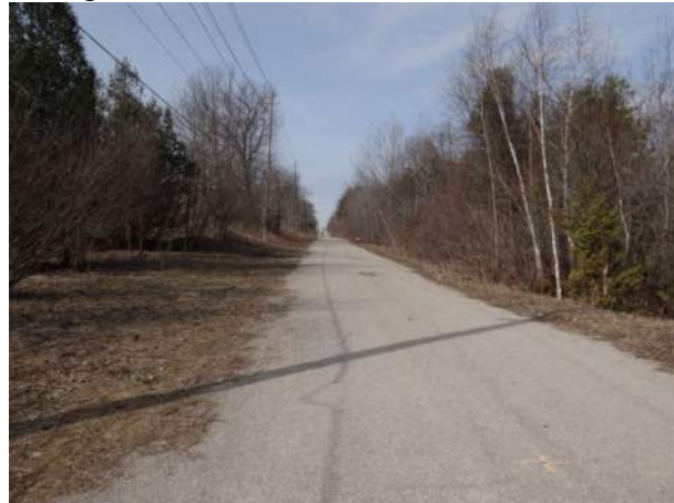
Plate 5: View across the intersection of the study area with Harvie Road, looking west.
