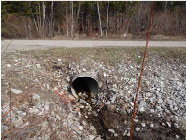
Plate 11: Looking north towards Harvie Road, across the westernmost two metal culvert.
