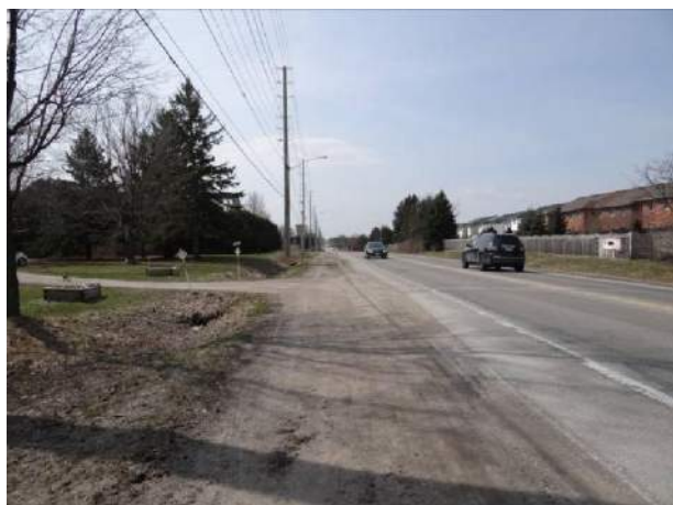
Plate 7: View south along Essa Road, trees on the east side obscure late twentieth-century residences from view, modern residential subdivision can be seen on the right (west) side.
