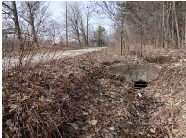
Plate 10: Concrete culvert located east of the reservoir, view west.
