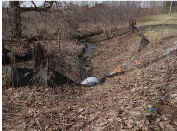
Plate 12: View south from the study area across the easternmost metal culvert.
