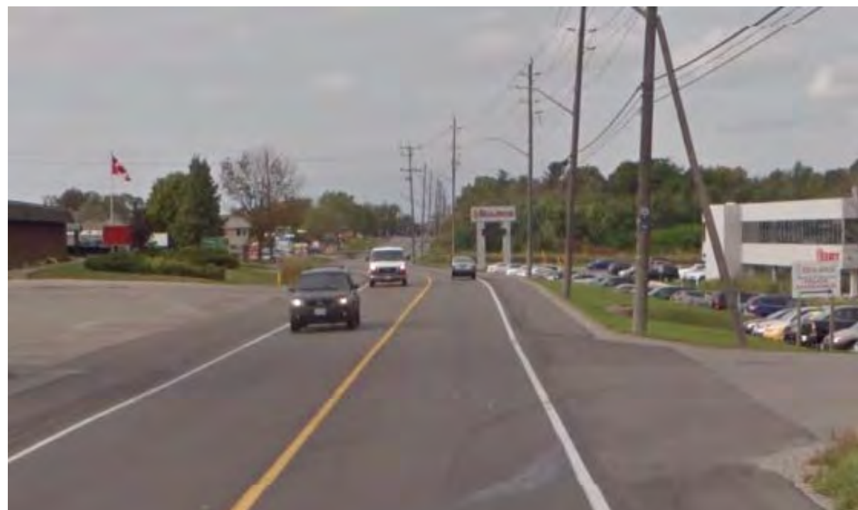
Looking north from The Source (south access)
