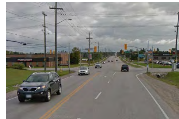
Big Bay Point Rd – looking E towards Huronia Rd
