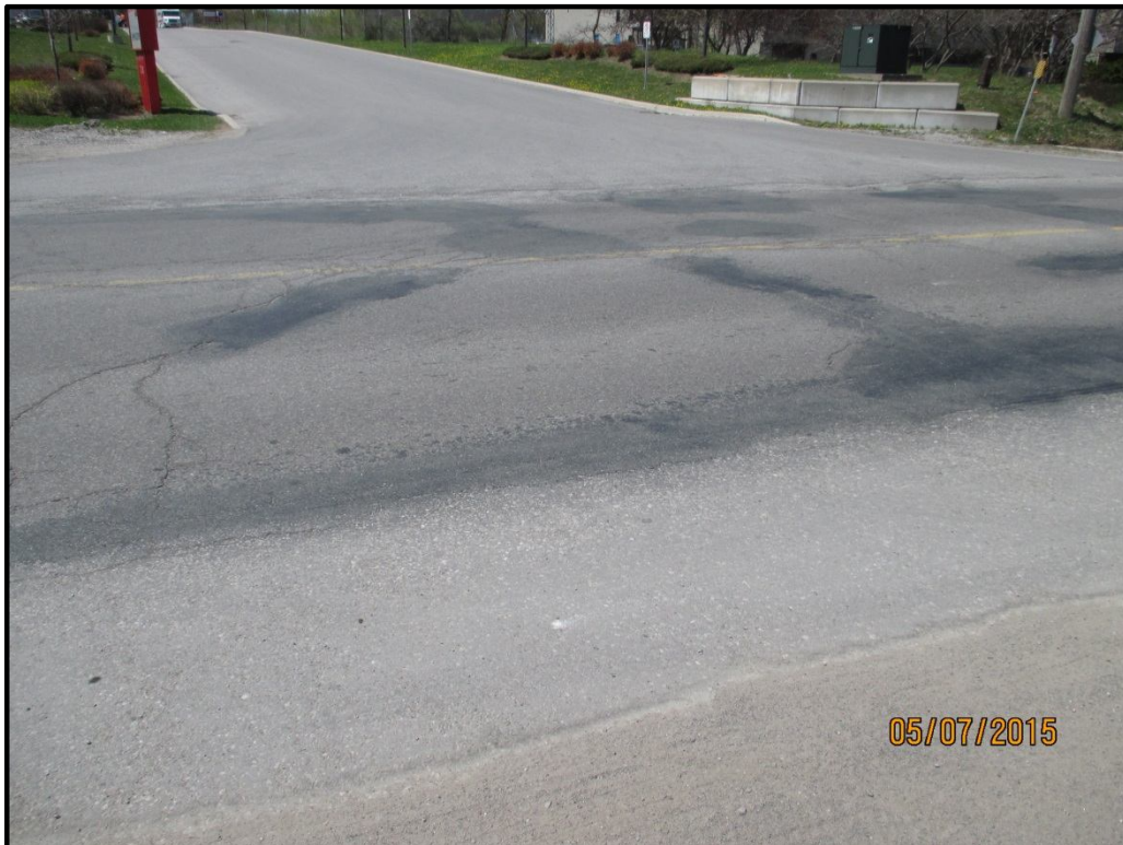
Cracks on Wearing Surface
