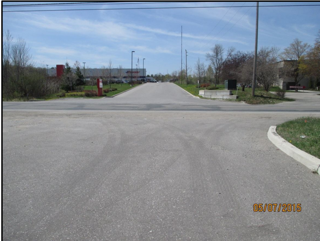
Roadway Looking West Over Culvert
