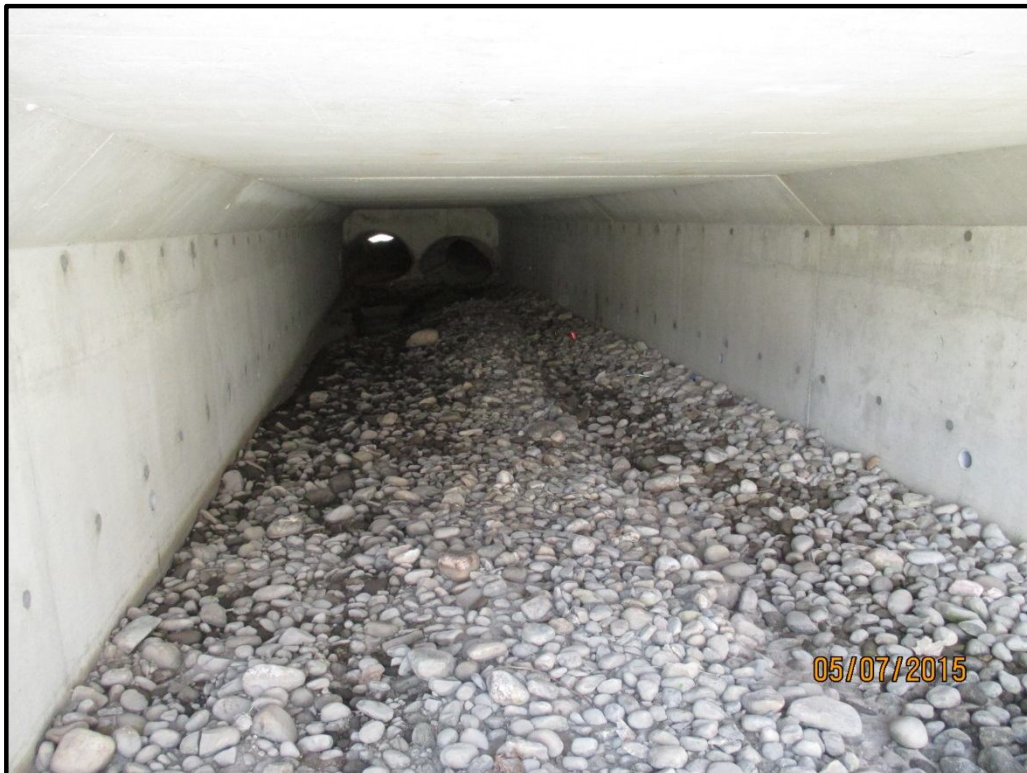
Concrete Barrel Looking South
