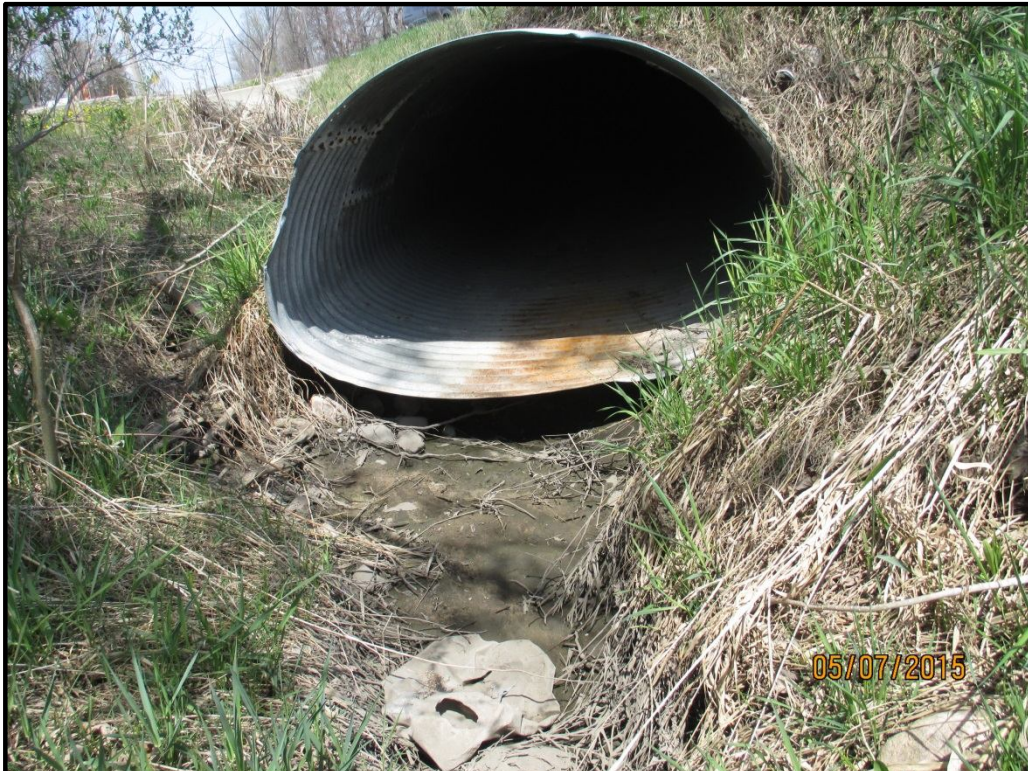
Undermining of Steel Barrels at South
