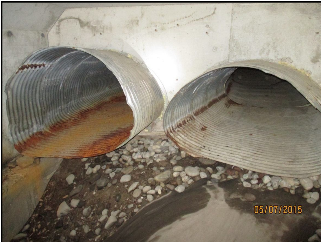
North Elevation of Steel Barrels
