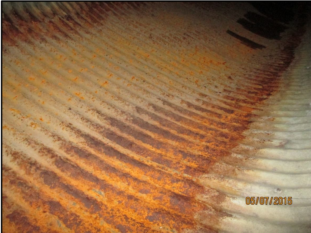
Surface Rusting at East Barrel Invert
