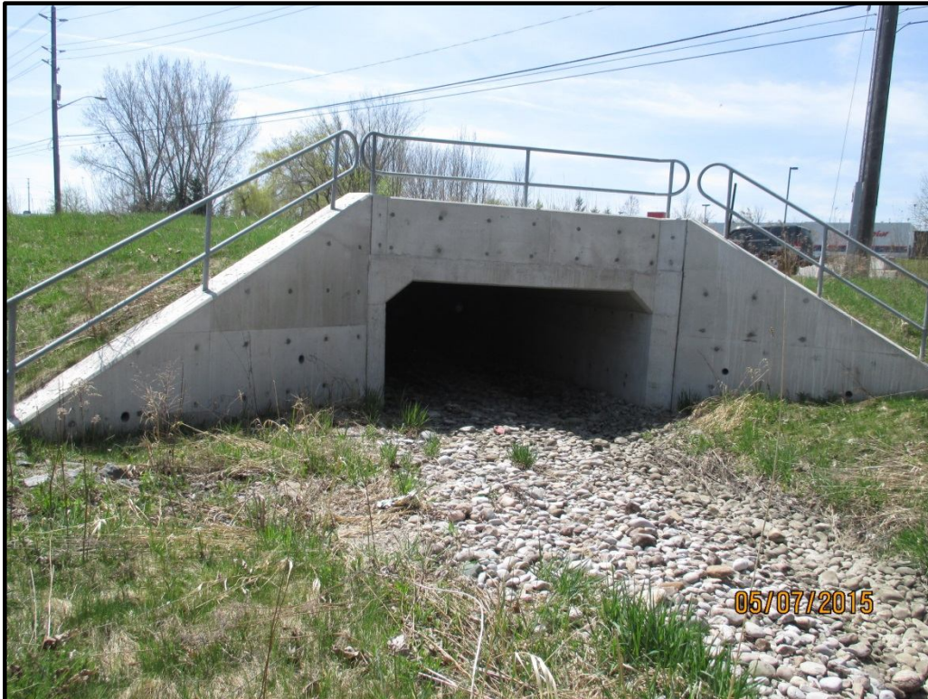
North Elevation of Concrete Culvert
