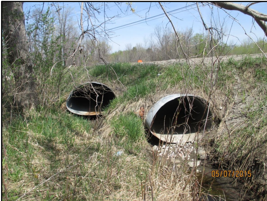
South Elevation of Steel Barrels
