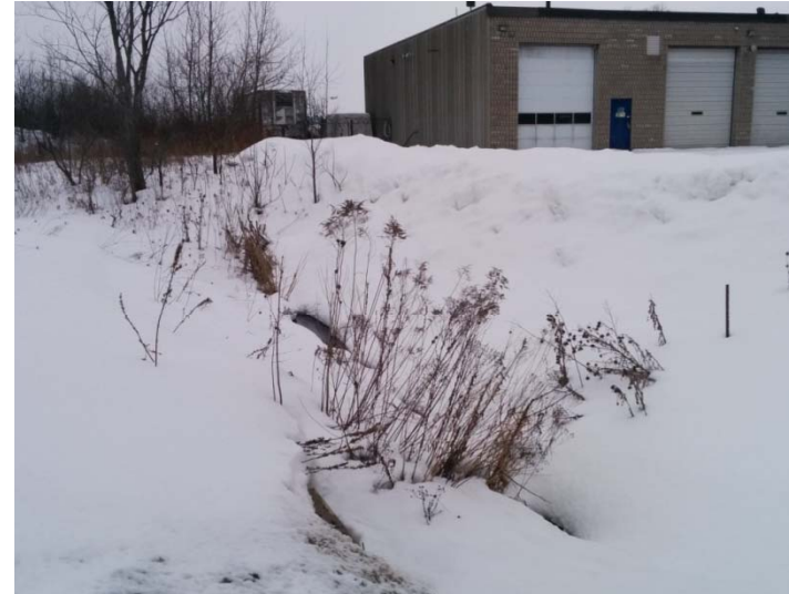
Photo 10: CR#2 – East side of Bayview Drive, southern exit. Existing structure (2016/01/27).
