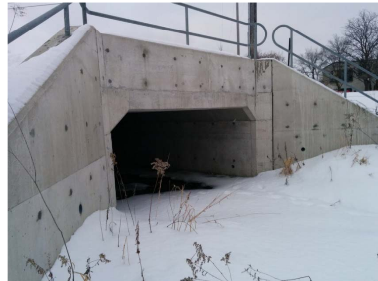
Photo 8: CR#2 – East side of Bayview Drive, northern exit. Existing structure (2016/01/27).
