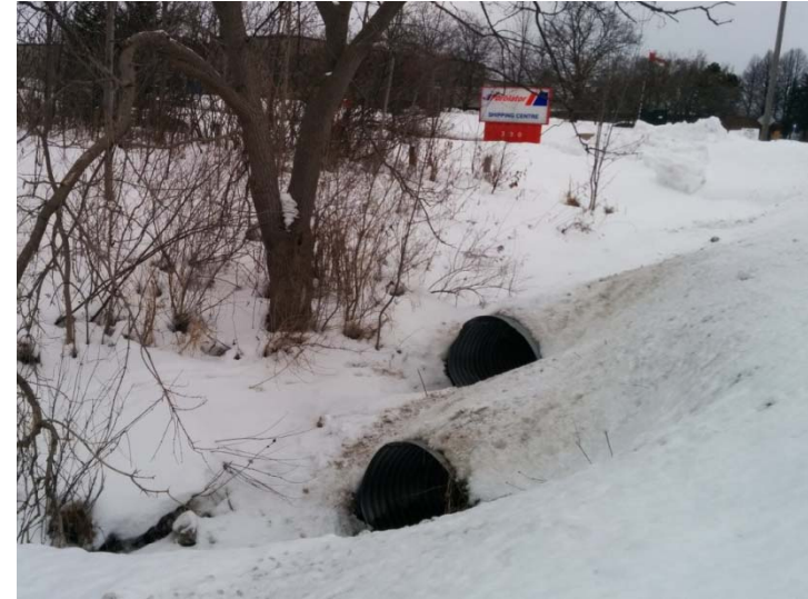
Photo 6: CR#2 – West side of Bayview Drive. Existing culverts (2016/01/27).
