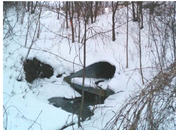
Photo 4: CR#1 – East side of Bayview Drive. Existing culvert (2016/01/27).
