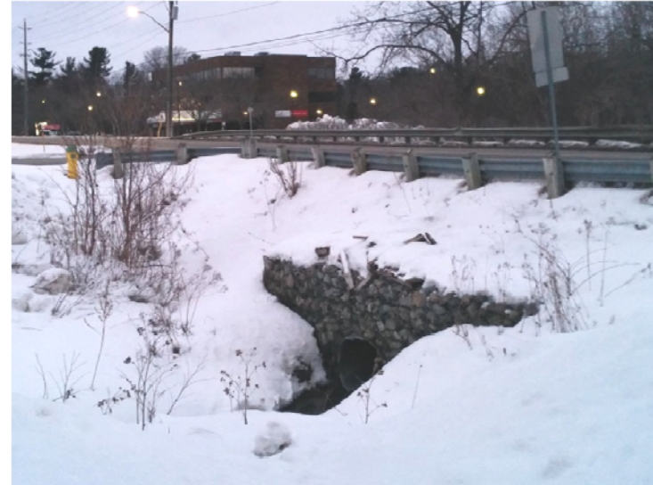
Photo 2: CR#1 - West side of Bayview Drive. Existing culvert (2016/01/27).
