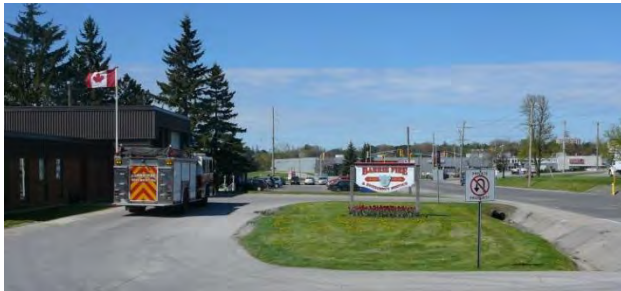
Photo 1: Barrie Fire Station 2
