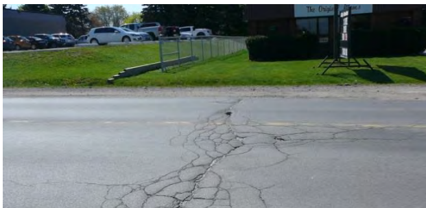
Photo 2: Existing Condition of Bell Farm Road
