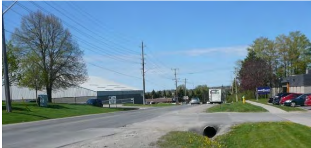
Photo 5: Existing Utilities on Bell Farm Road
