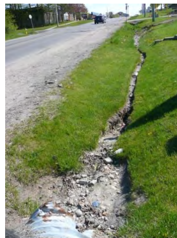
Photo 4: Ditches along Bell Farm Road
