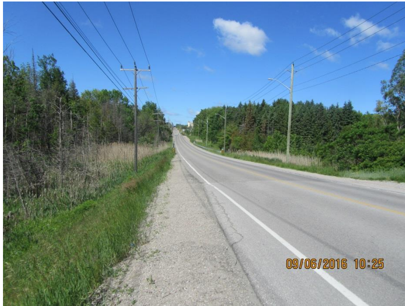
Photograph No. 7: Lockhart Road east of Huronia Rd approximately 0.34km; facing west
