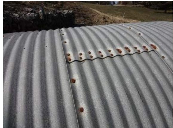
#6 – Rusted Bolts Appears to be non-galvanized
