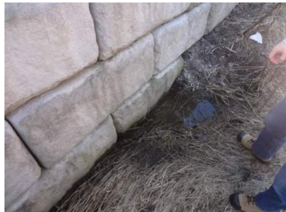
#6 – Excessive Water Seeping through the Retaining Wall
