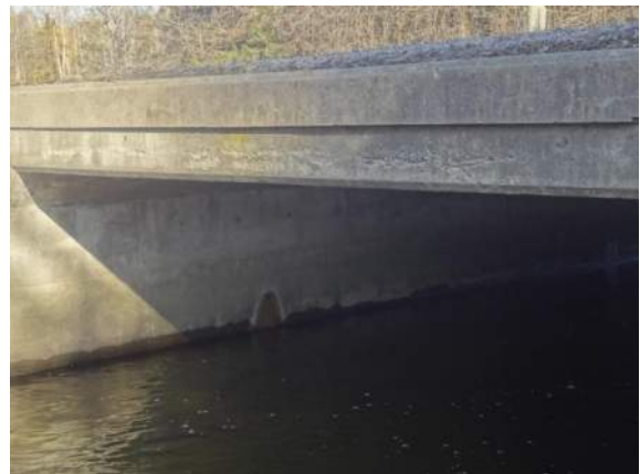
#6 – Observed Spalling at Top Slab
