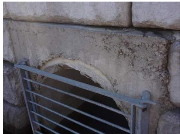
#6 – Buckling and Spalling at Storm Sewer Outlets
