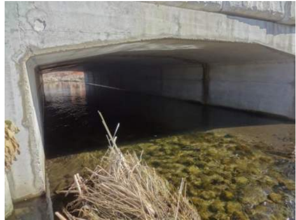
#6 – Buckling and Spalling at Storm Sewer Outlets
