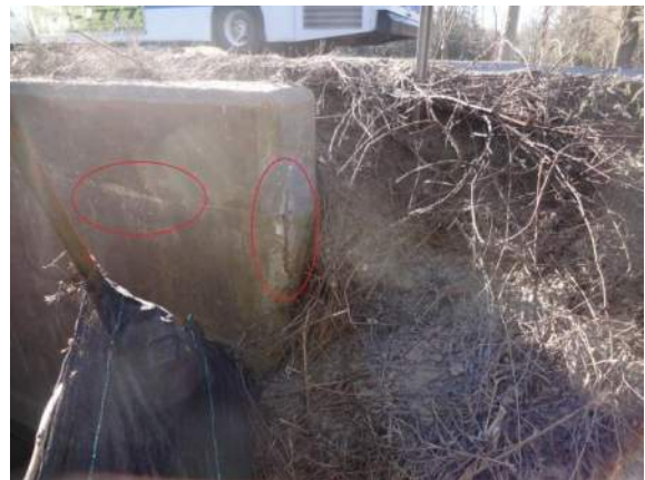
#6 – Observed Spalling at Top Slab
