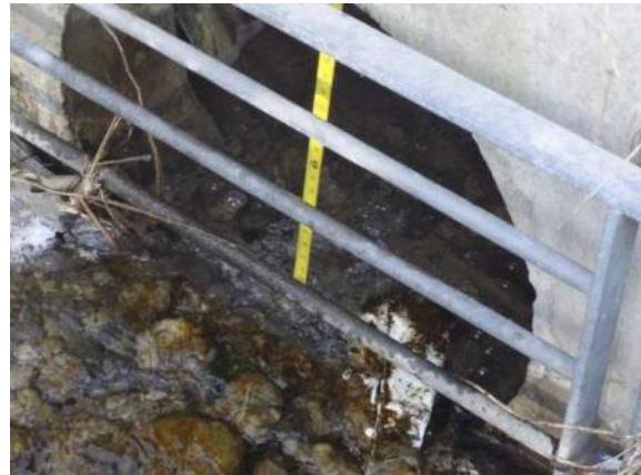
#6 – Excessive Water Seeping through the Retaining Wall
