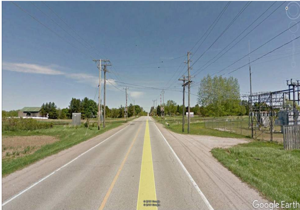
Figure 2: Looking east along Lockhart Road toward existing level crossing.
